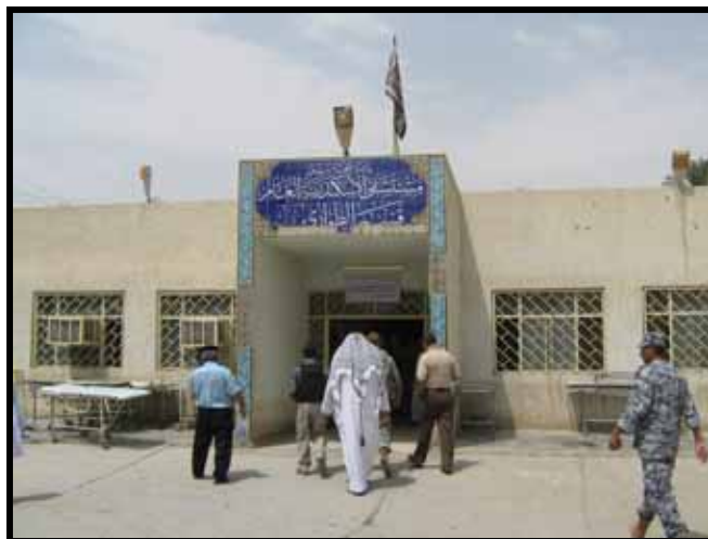
Emergency Care Facility
